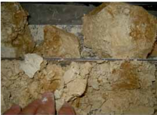
Moderately to heavily stained and clay-filled joints (open > 3mm) CIRIA grade C and orange-stained softened chalk
