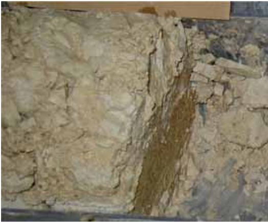
Moderately stained and polished sub-horizontal joint (open < 3mm) CIRIA grade B and orange-stained chalk
