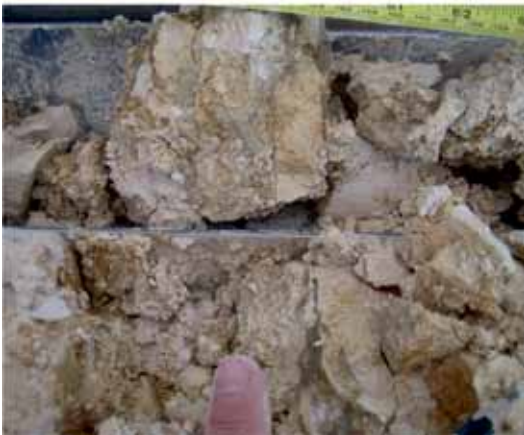
Moderately to heavily stained and clay-filled joints (open > 3mm) CIRIA grade C and orange-stained and softened chalk
