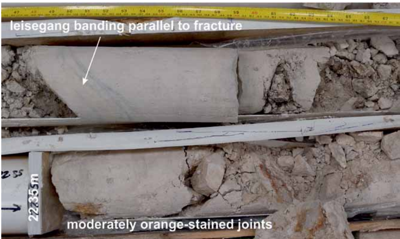
Figure C5a12 Moderately stained 'slightly open' joints, CIRIA grade B, and dirt-filled open joints, grade C. Liesegang banding internally in the chalk is parallel to a fracture (indicating groundwater movement).
